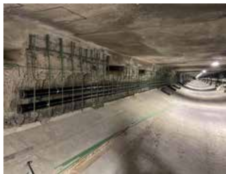
The 15,000v cables and conduit wall had to be replaced.
